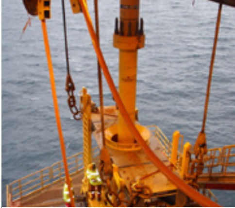
View of riser through the Texas deck
